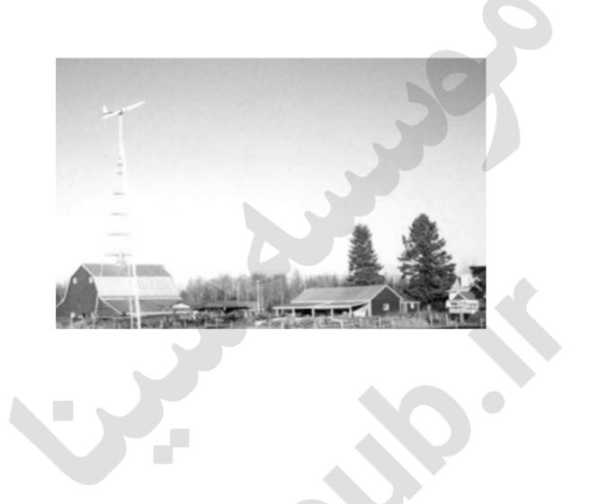
In Clover Valley, Minnesota, this 3-kW Whisper H175 turbine on a 50-foot tower is connected to the utility grid to offset the farm's utility-supplied electricity
