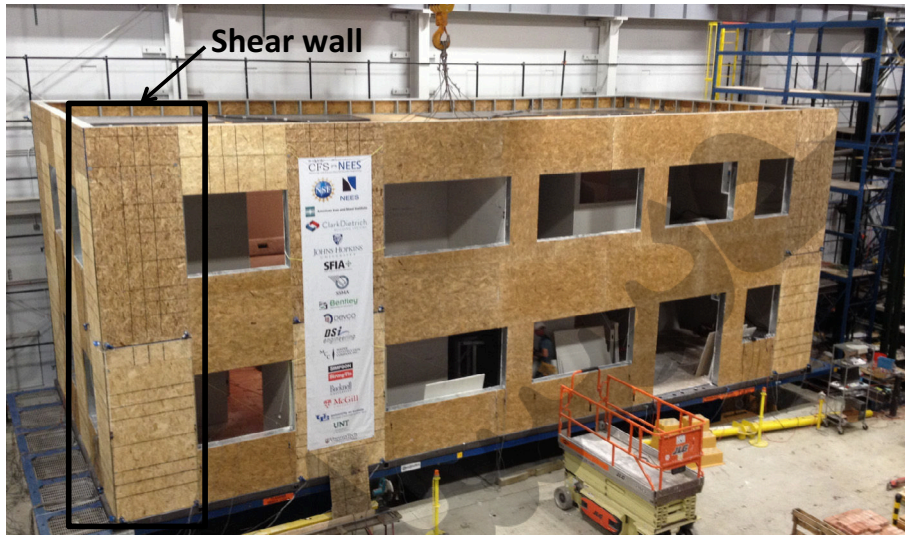
Fig. 1. CFS-NEES building and shear wall in it.
